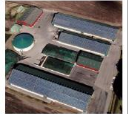
System power: 668,76 kWp
